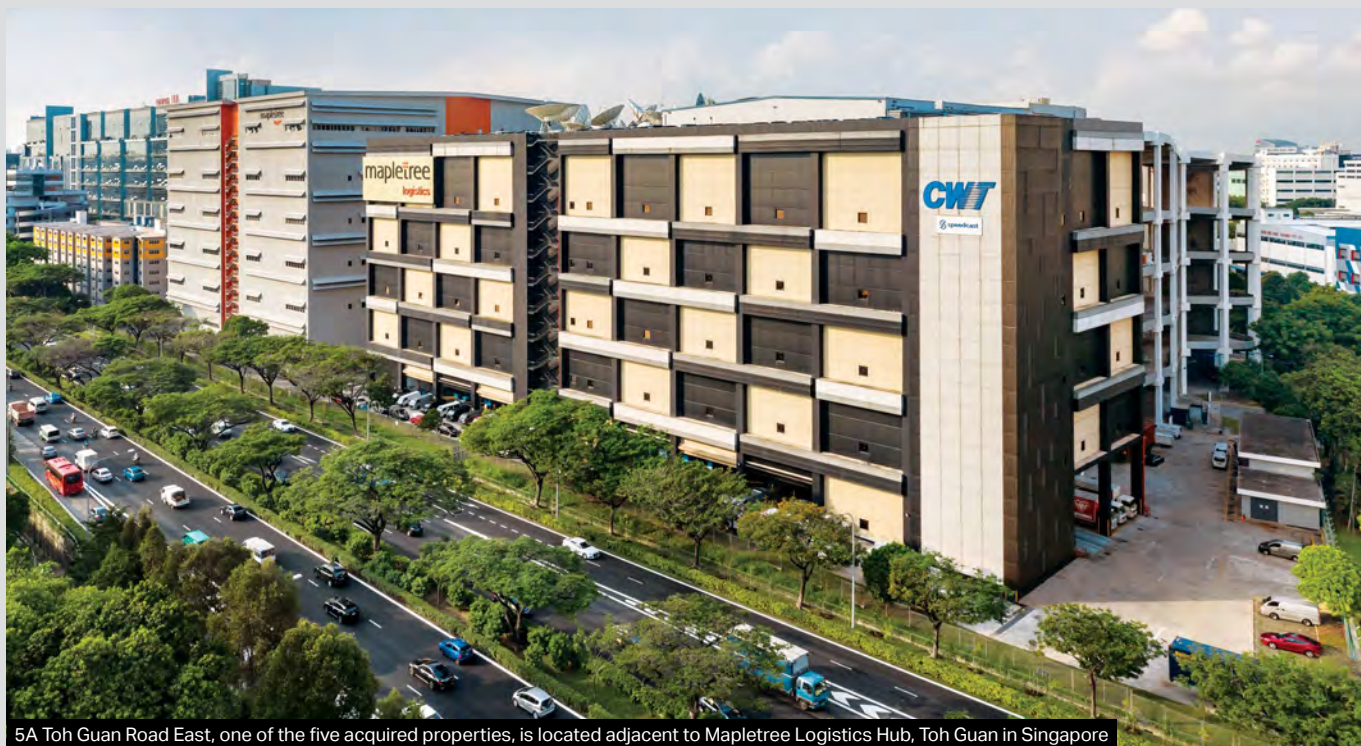
5A Toh Guan Road East, one of the five acquired properties, is located adjacent to Mapletree Logistics Hub, Toh Guan in Singapore
