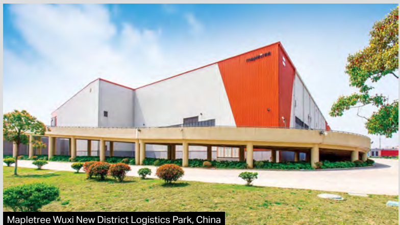
Mapletree Wuxi New District Logistics Park, China
