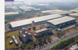
Mapletree Logistics Park Talegaon
