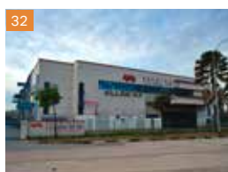
30 Tuas South Avenue 8
