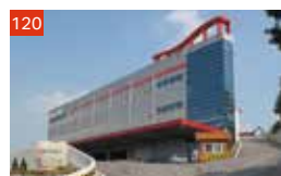
Mapletree Logistics Centre – Hobeob 1
