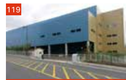
Mapletree Logistics Centre – Majang 1
