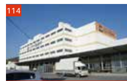
Mapletree Logistics Centre – Anseong Cold
