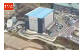
Mapletree Logistics Centre – Majang 2
