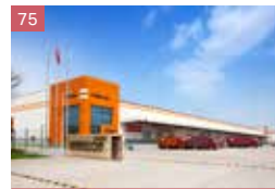
75 Mapletree Nantong Chongchuan Logistics Park
