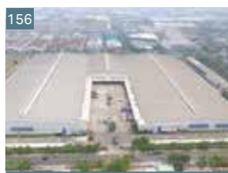
Unilever VSIP Distribution Centre
