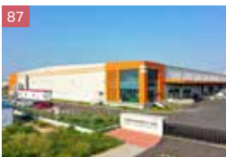
87 Mapletree Tianjin Xiqing Logistics Park
