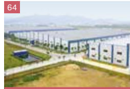
64 Mapletree American Industrial Park
