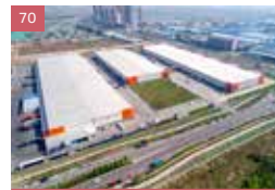
70 Mapletree Fengdong (Xi'an) Industrial Park
