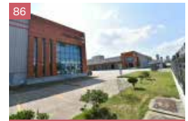
86 Mapletree Nantong (EDZ) Logistics Park
