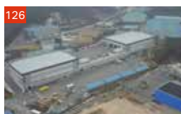
Mapletree Logistics Centre – Hobeob 3
