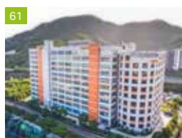
Mapletree Logistics Hub Tsing Yi
