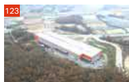
Mapletree Logistics Centre – Iljuk 2
