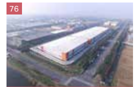
76 Mapletree Hangzhou Logistics Park
