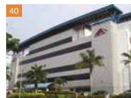
15 Changi South Street 2
