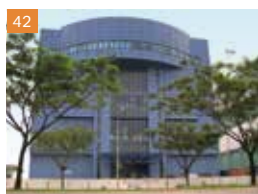
73 Tuas South Avenue 1
