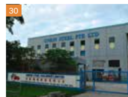
31 & 33 Pioneer Road North
