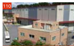
Mapletree Logistics Centre – Yeosu
