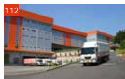
Mapletree Logistics Centre – Iljuk
