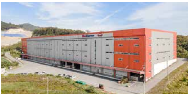
Mapletree Logistics Centre - Iljuk 2
