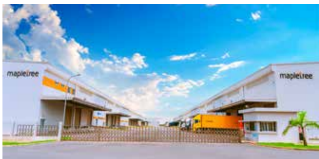
Mapletree Logistics Park Bac Ninh Phase 3
