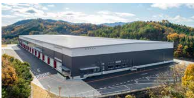
Higashi Hiroshima Centre
